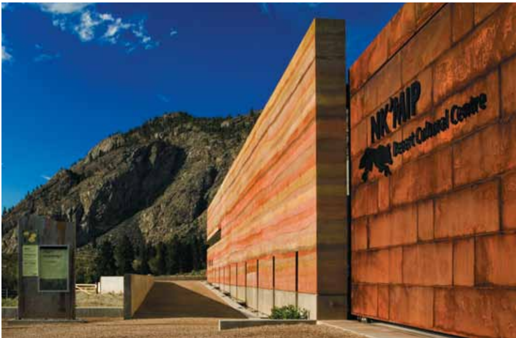
NK'MIP Desert Cultural Centre, Osoyoos, British Columbia Hotson Bakker Boniface Haden Architects + Urbanistes PHOTO: NIC LEHOUX
